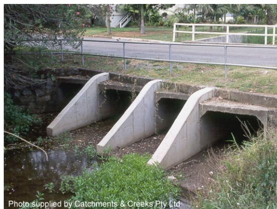
Figure 6.6.3. Debris Deflector Walls
