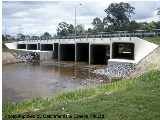
Figure 6.6.6. Multi-Cell Culvert with Different Invert Levels
