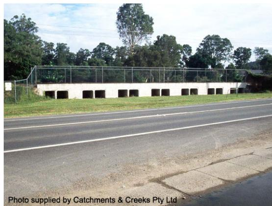
Figure 6.6.2. Floodplain Culvert
