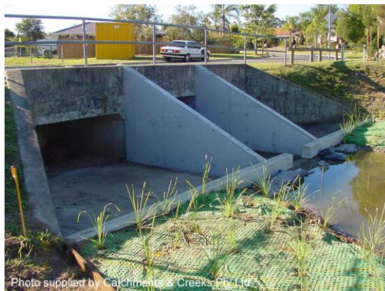
Figure 6.6.7. Debris Deflector Walls and Sediment Training Wall Added to Existing Culvert
