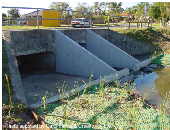
Figure 6.6.7. Debris Deflector Walls and Sediment Training Wall Added to Existing Culvert
