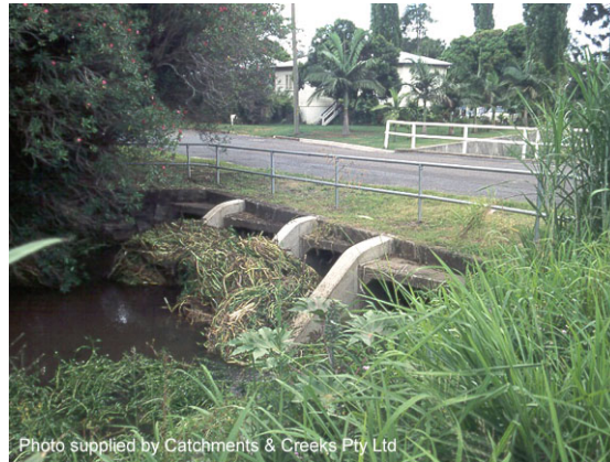
Figure 6.6.4. Post Flood Collection of Debris on Top of Deflector Walls
