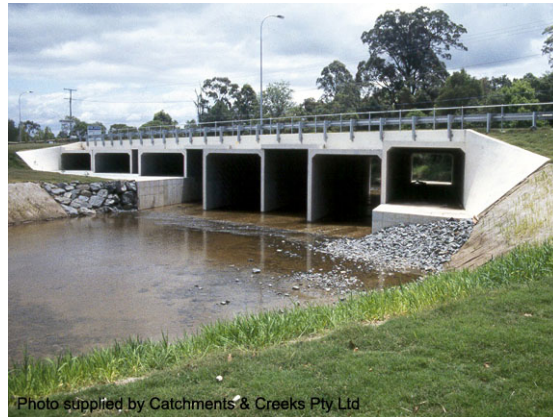
Figure 6.6.6. Multi-Cell Culvert with Different Invert Levels
