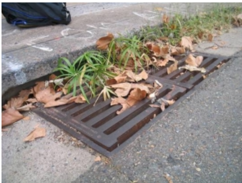
Figure 2.12: Vegetation growing in inlet indicates poor maintenance
