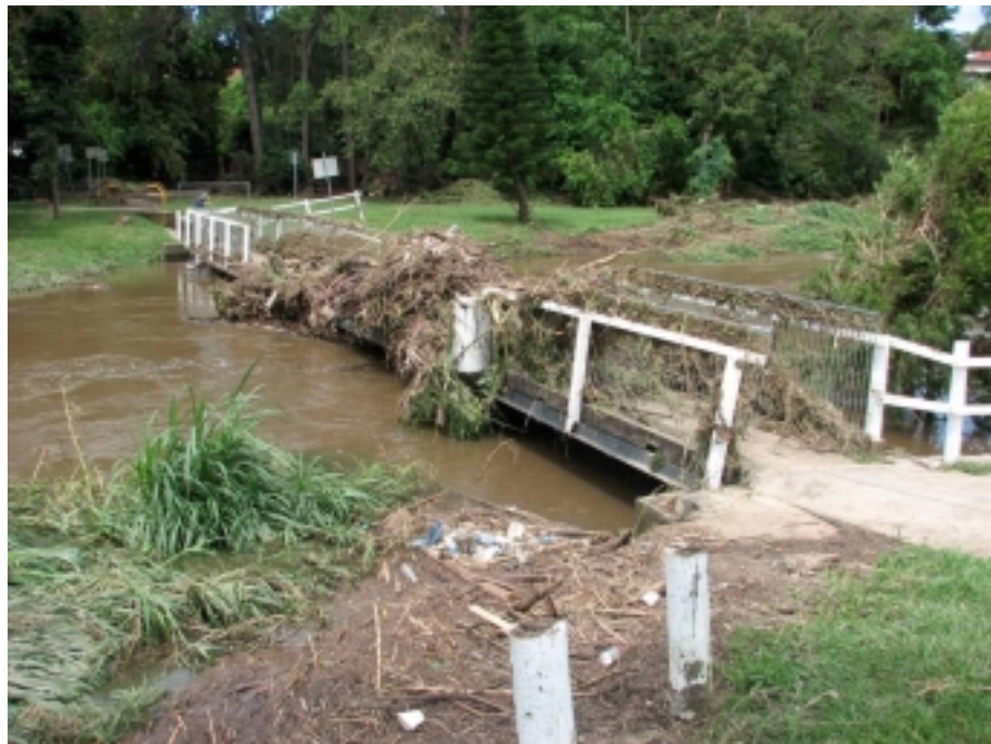
Figure 2.13: Guardrails on a bridge can collect debris
