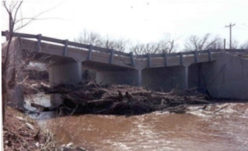
Figure 3.4 – Debris Accumulation Bridge Failure
