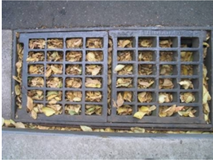
Figure 2.9: Leaves can completely block inlets
