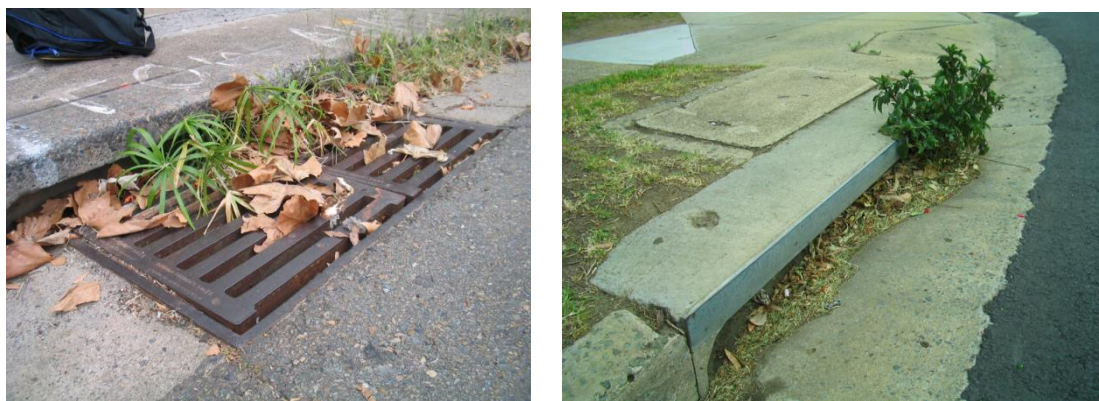
Photo 21: Poor Pit Maintenance
