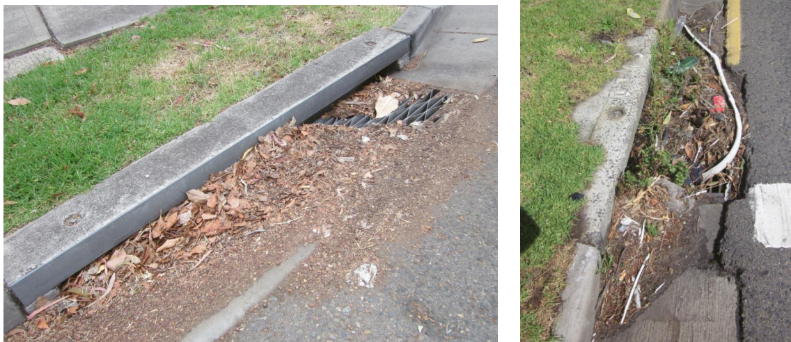
Photo 18: Examples of Kerb Inlet Pit Blockages, Sydney
