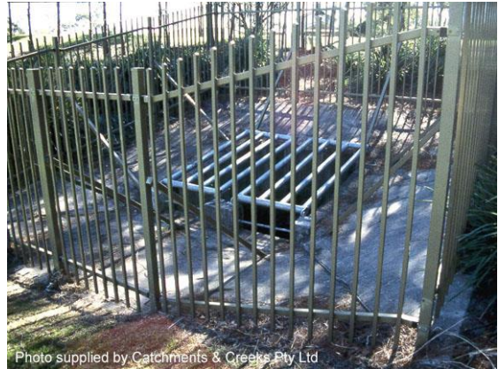
Photo 23: Safety screen surrounding screened detention basin outlet
