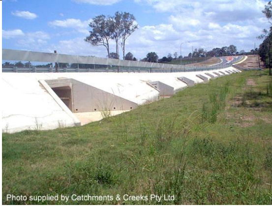
Photo supplied by Catchments & Creeks Pty Ltd Photo 28: Series of floodplain culverts
