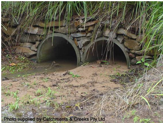
Photo 4: Sediment blockage of stormwater pipes
