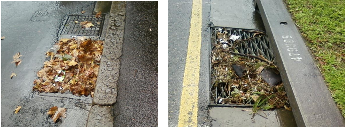
Photo 17: Examples of Grated Pit Blockages, Sydney
