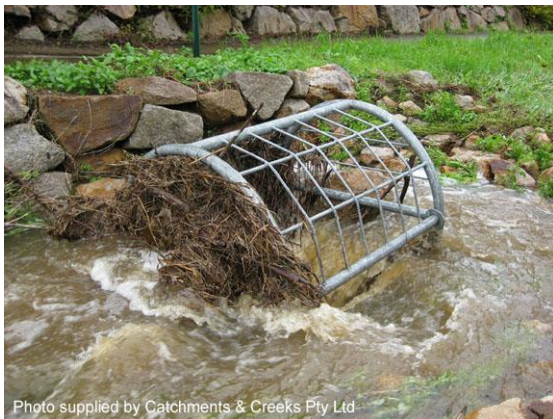
Photo 24: Dome inlet screen with minor blockage
