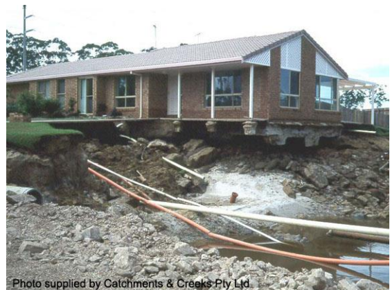
Photo 9: House adjacent to culvert (left) undermined by flows bypassing the culvert
