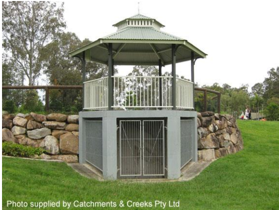
Photo 26: Detention basin outlet chamber
