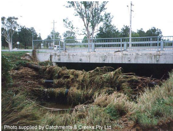
Photo supplied by Catchments & Creeks Pty Ltd Photo 12: Debris collected around exposed pipes
