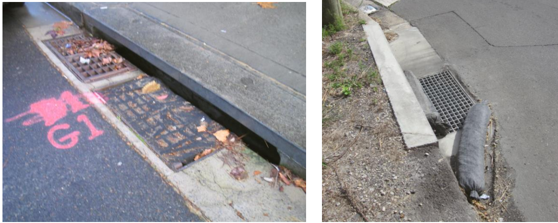
Photo 19: Deliberate Blockages for Sediment and Erosion Control
