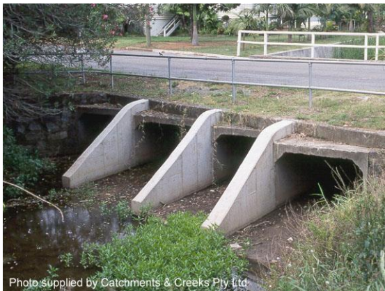
Photo supplied by Catchments & Creeks Pty Ltd Photo 30: Debris deflector walls
