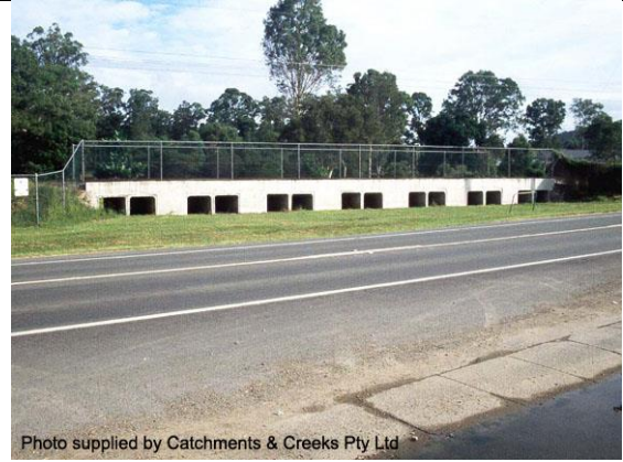
Photo supplied by Catchments & Creeks Pty Ltd Photo 29: Floodplain culvert
