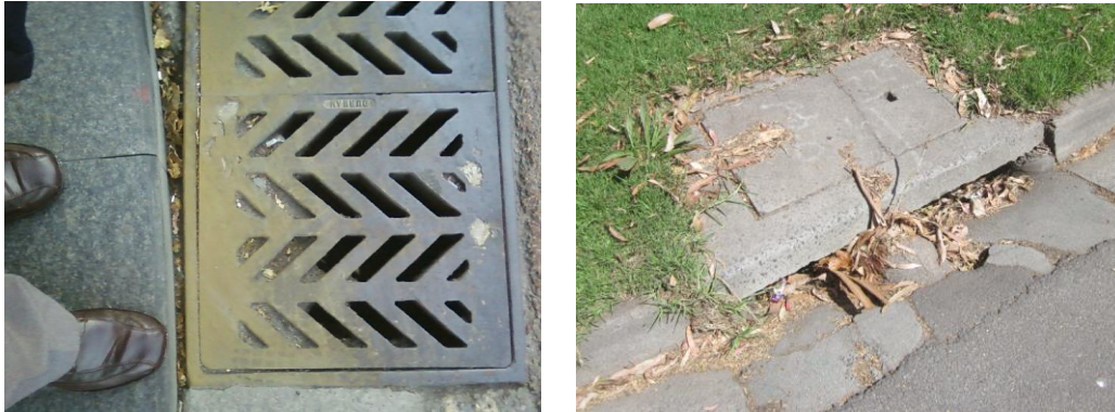
Photo 16: Examples of Pit Blockages, Sydney and Melbourne
