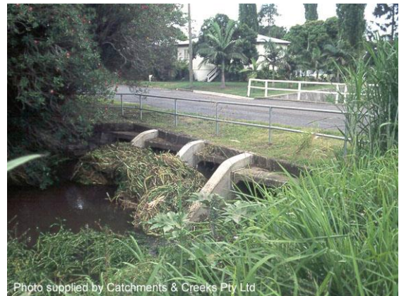
Photo supplied by Catchments & Creeks Pty Ltd Photo 31: Post flood collection of debris on top of deflector walls
