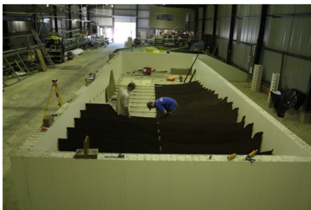
Figure 13: Template Installation
